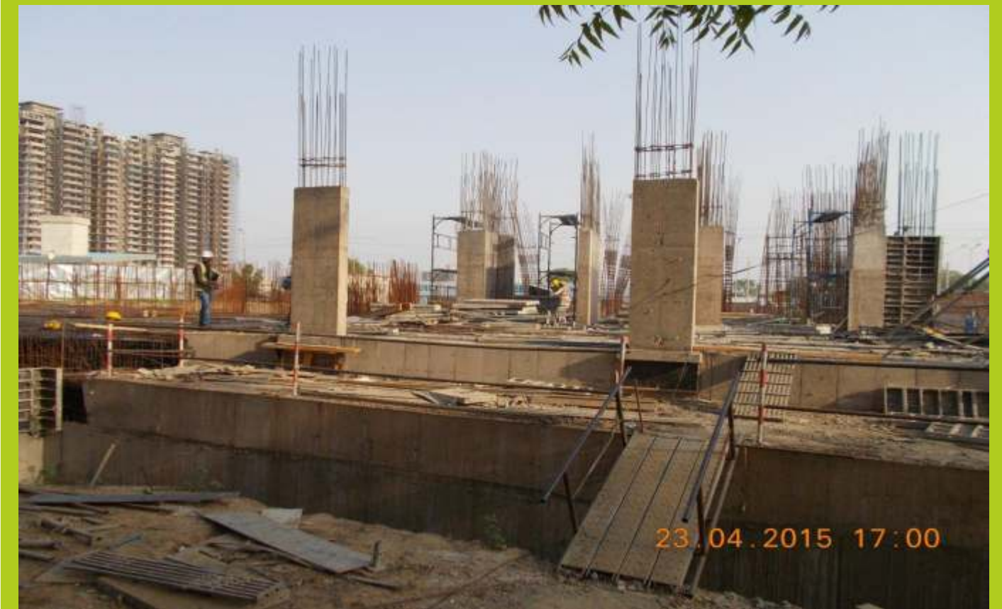
TOWER A April 2015 Ground Floor slab 50% completed
