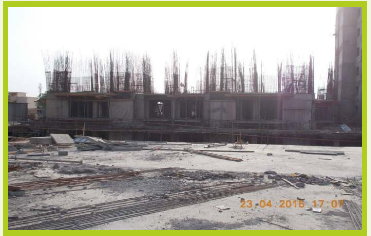
TOWER C April 2015 1st floor slab 67% completed
