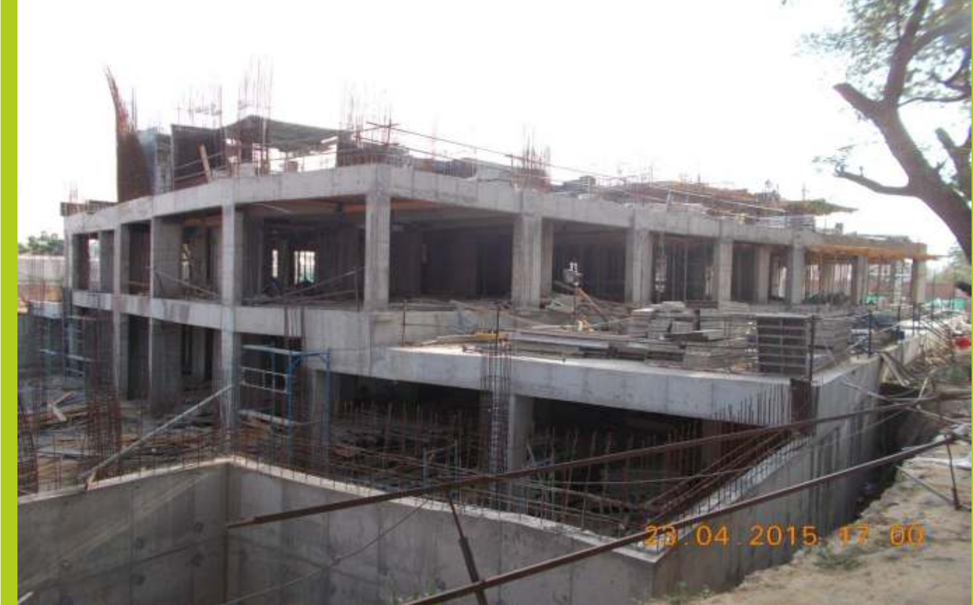
TOWER B April 2015 2nd floor slab 50% completed
