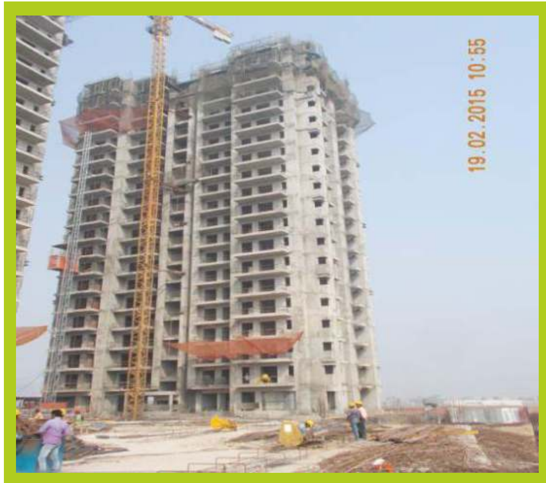
TOWER H February 2015 20th floor slab completed
