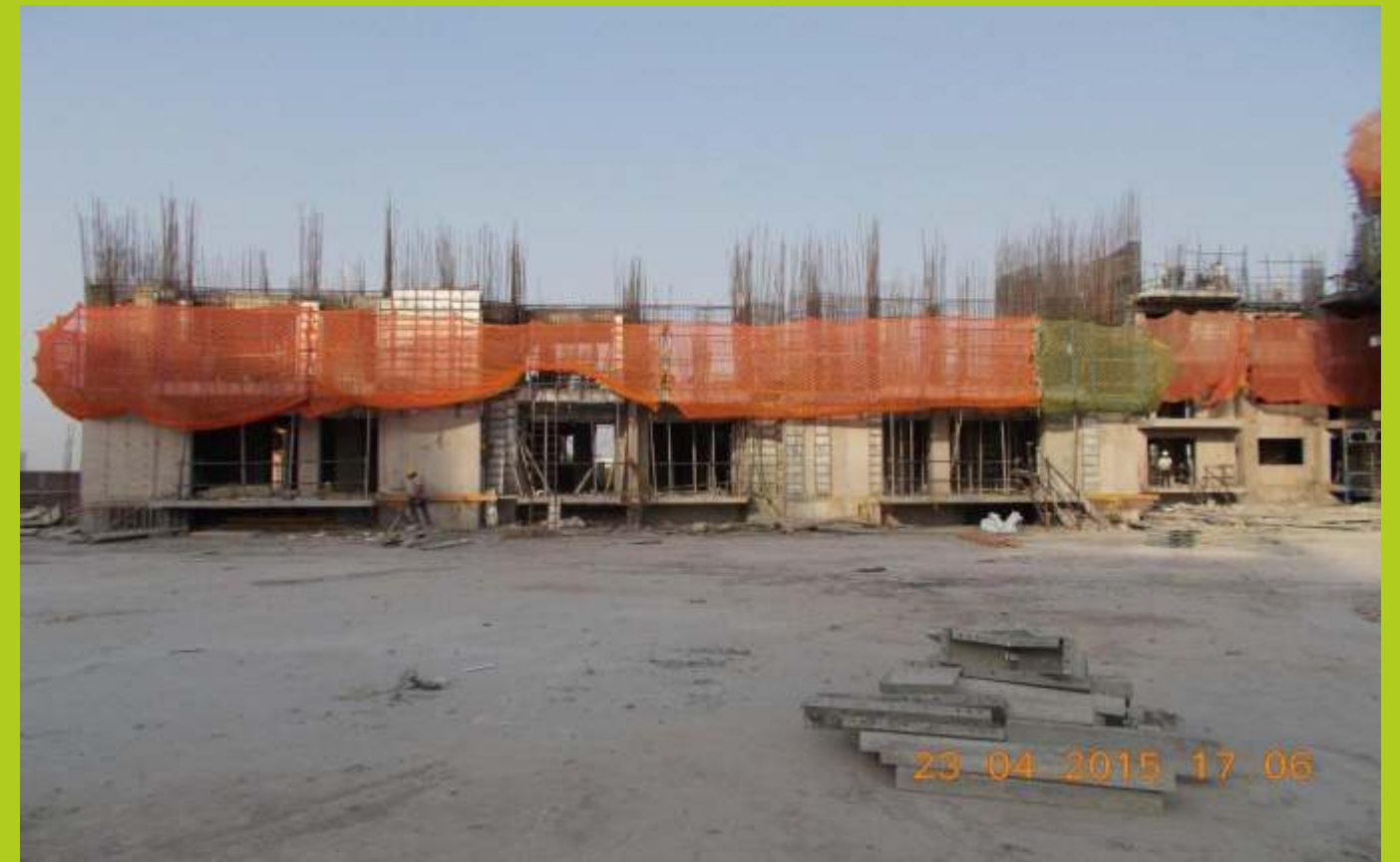
TOWER K April 2015 1st floor slab 67% completed
