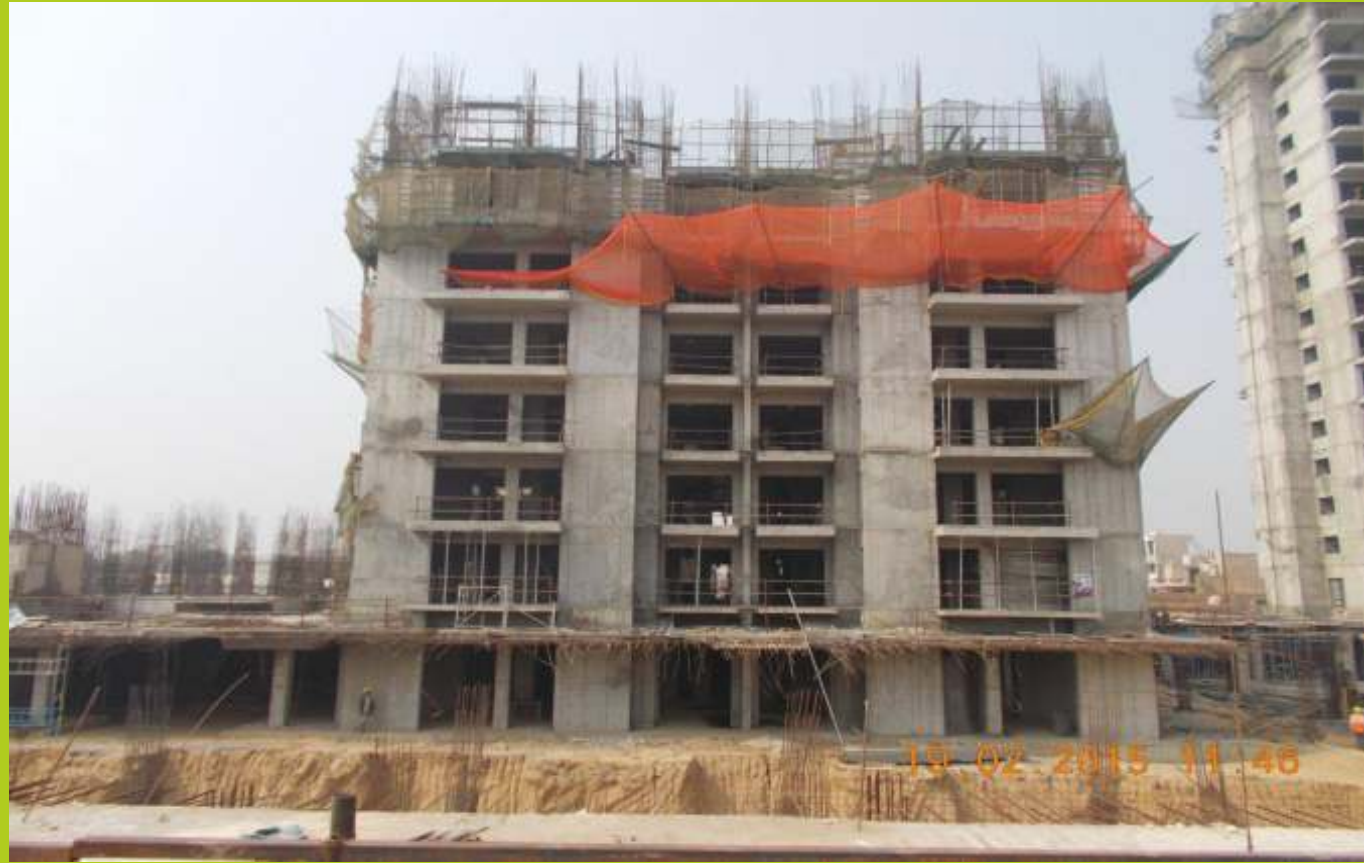
TOWER D February 2015 6th floor slab completed
