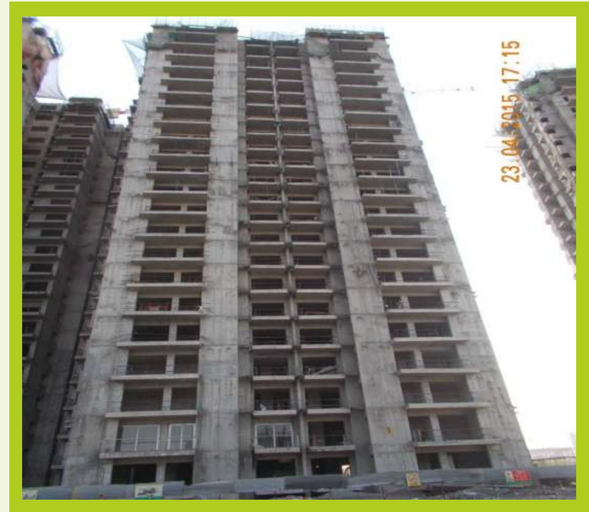
TOWER F April 2015 Super structure completed Plaster work under progress
