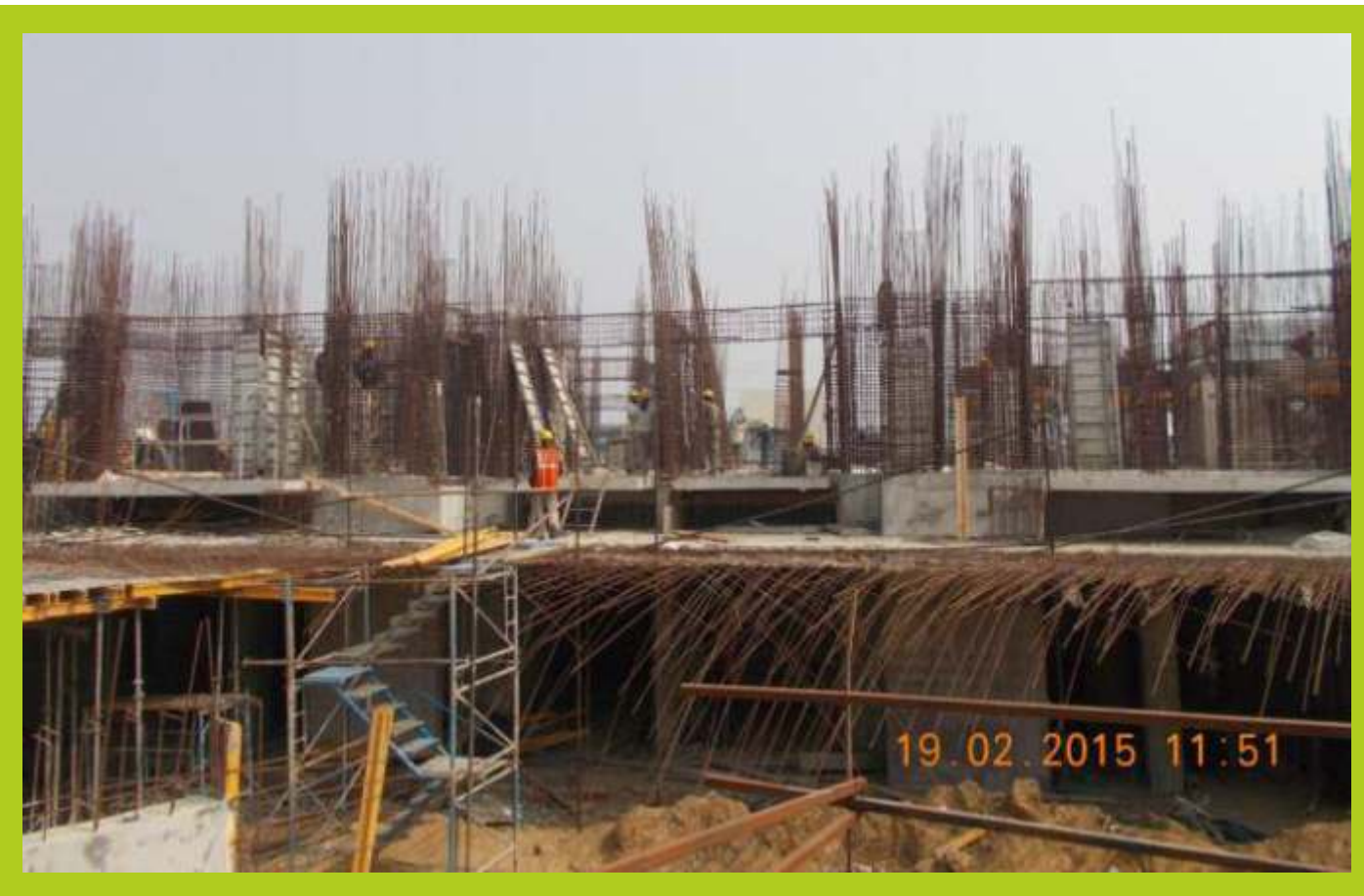
TOWER L February 2015 Ground floor slab completed
