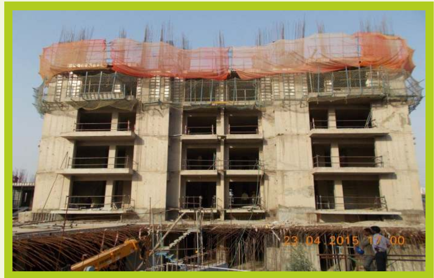
TOWER L April 2015 4th floor slab 35% completed
