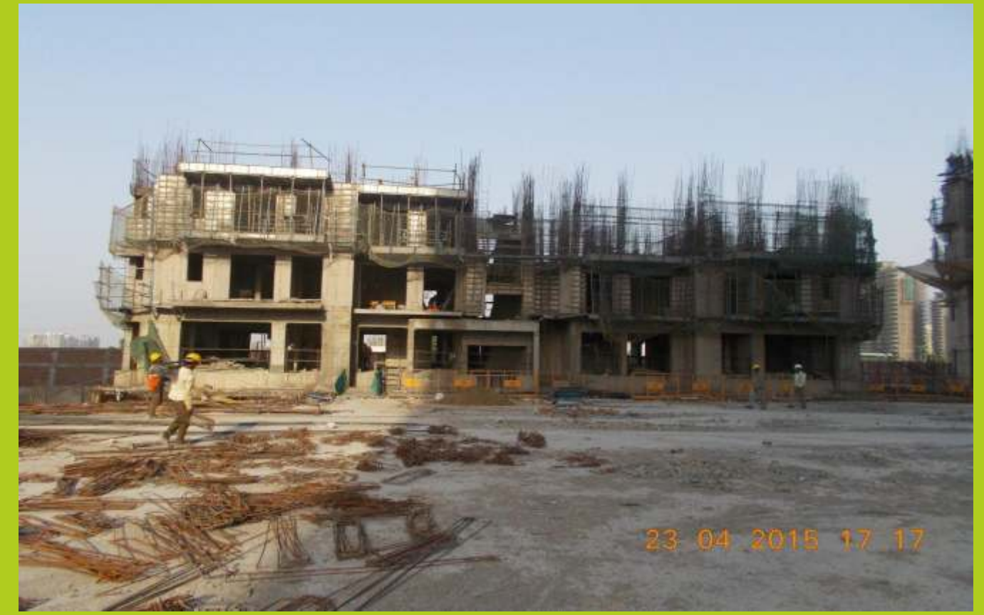
TOWER I April 2015 2nd floor slab completed
