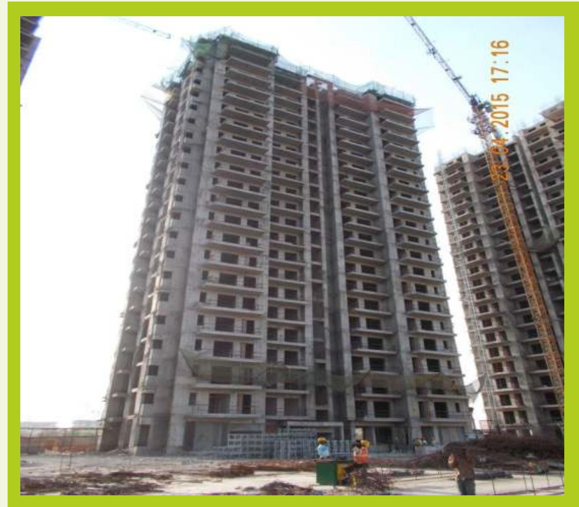
TOWER G April 2015 Super structure completed Plaster work under progress
