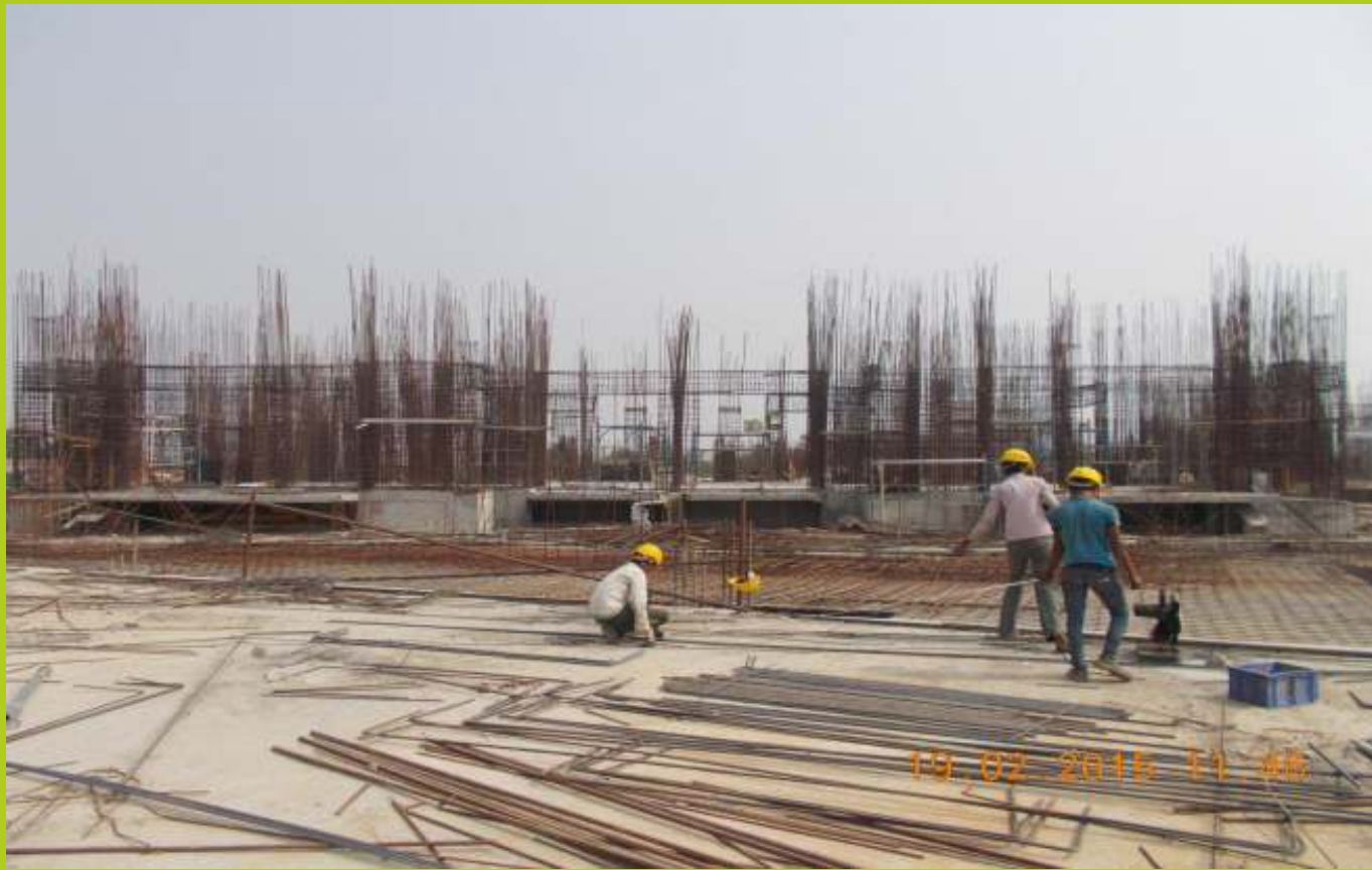
TOWER K February 2015 Ground floor slab completed
