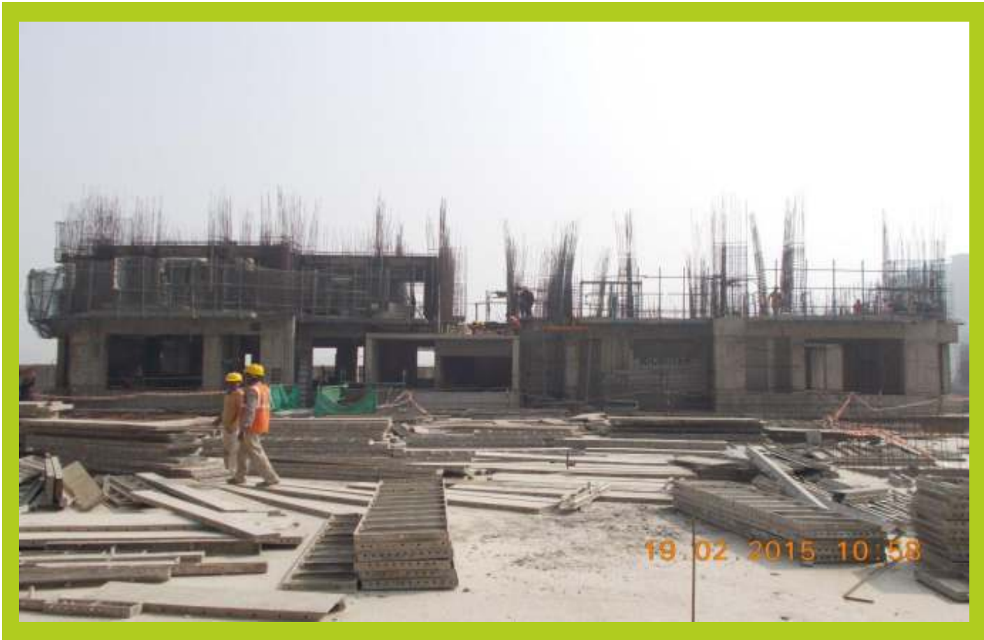
TOWER J February 2015 1st floor slab completed
