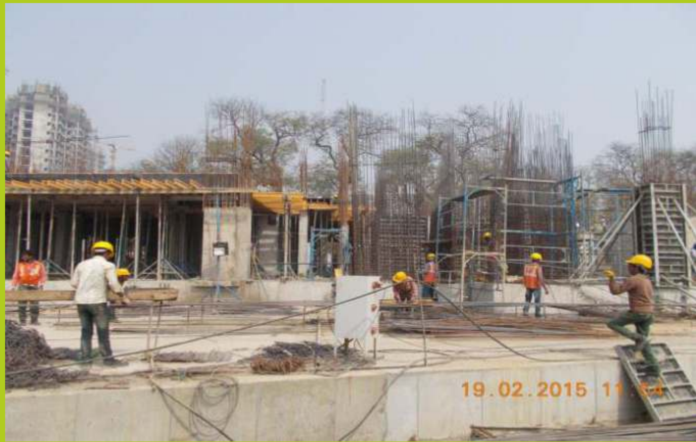
TOWER B February 2015 Ground floor slab completed
