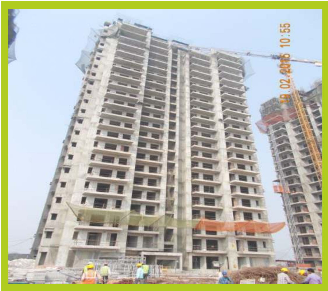
TOWER G February 2015 Super structure completed
