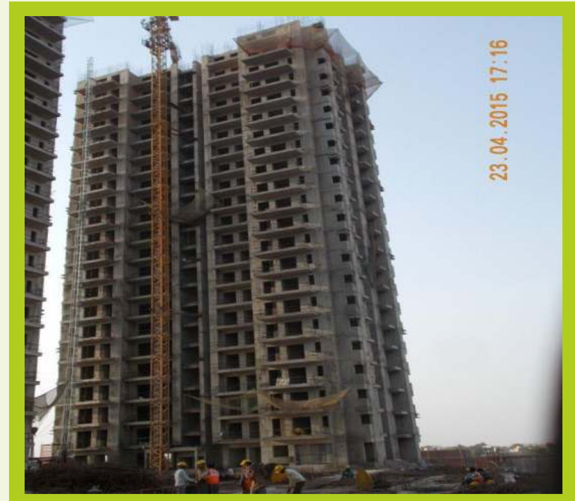
TOWER H April 2015 Super structure completed Plaster work under progress
