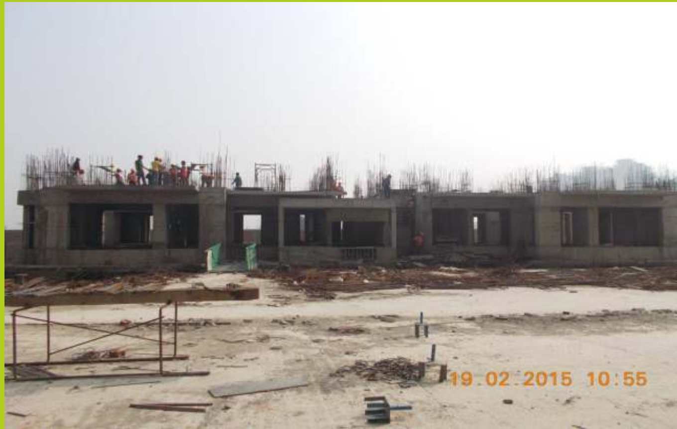
TOWER I February 2015 1st floor slab completed
