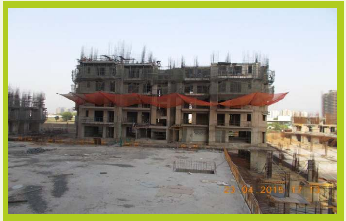
TOWER J April 2015 4th floor slab completed
