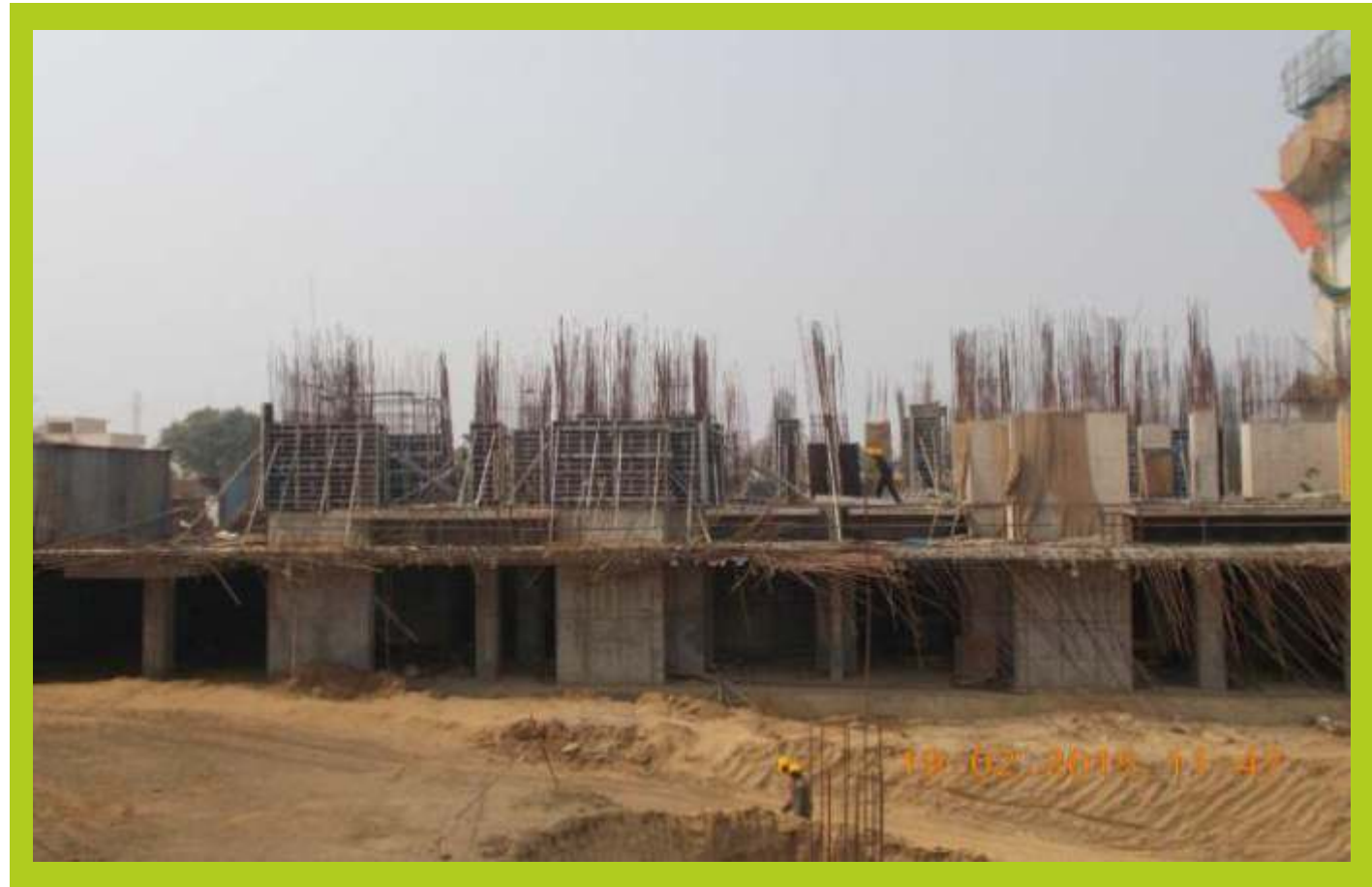
TOWER C February 2015 Ground floor slab completed
