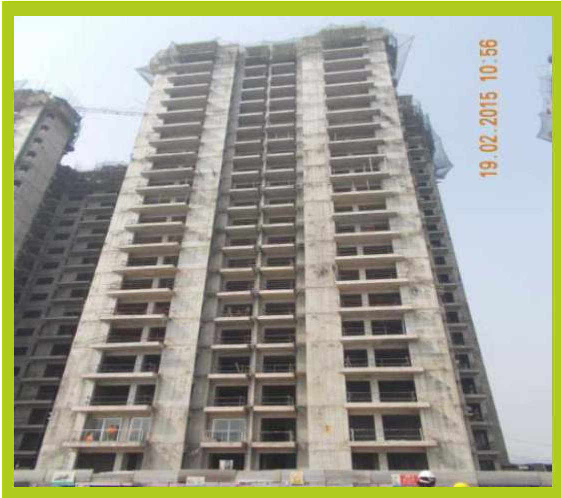
TOWER F February 2015 Super structure completed
