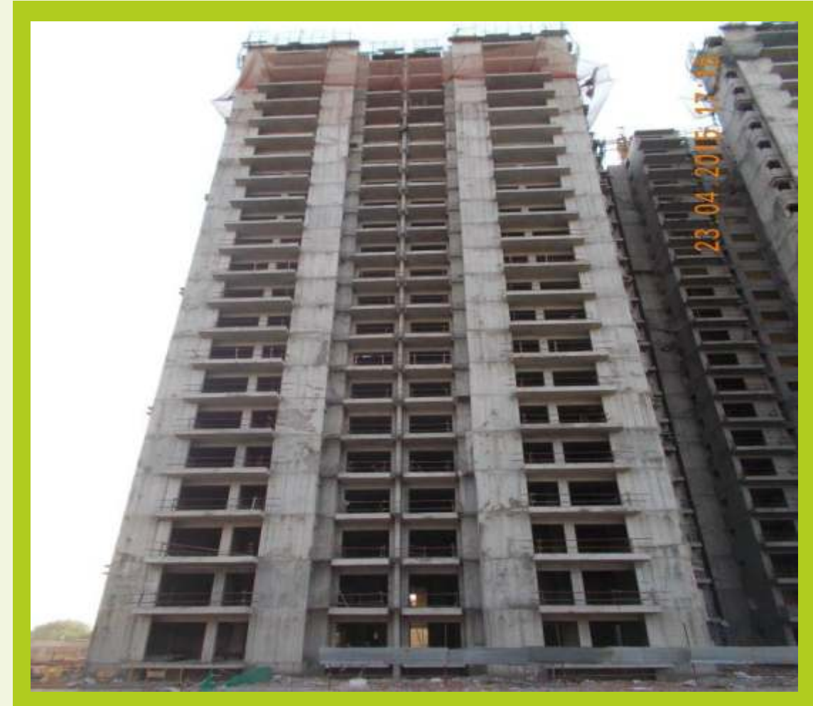
TOWER E April 2015 Super structure completed Plaster work under progress
