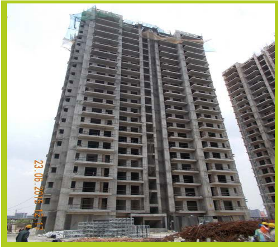
TOWER G June 2015 Super structure completed Interior plaster work under progress
