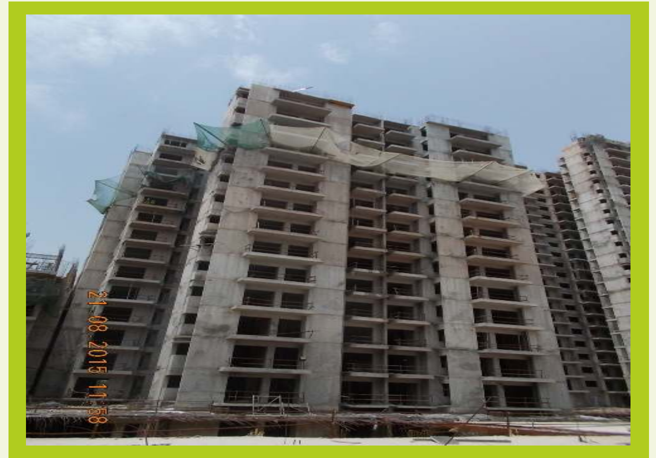
TOWER D August 2015 Super Structure completed Interior plaster work under progress
