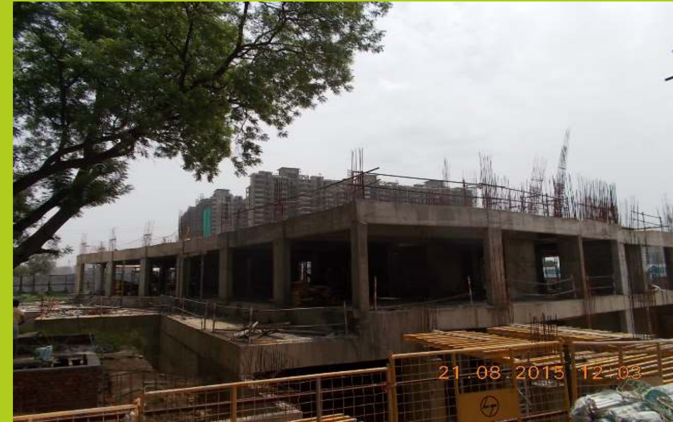
TOWER A August 2015 Ground floor slab 80% completed 1st floor slab 40% completed
