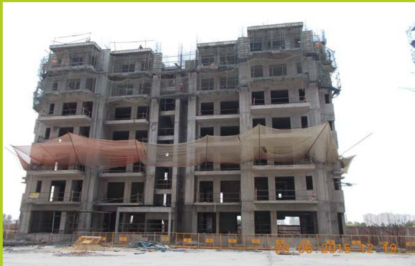
TOWER I June 2015 7th floor slab 50% completed
