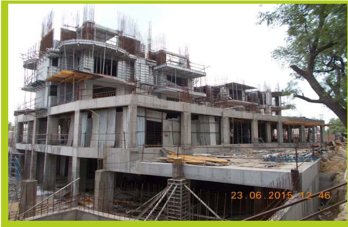
TOWER B June 2015 3rd floor slab 50% completed
