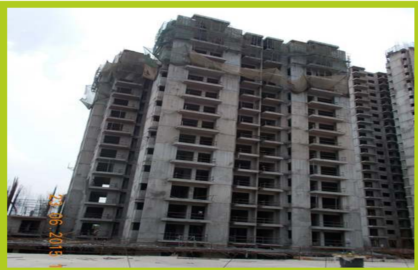
TOWER D June 2015 Terrace floor slab casted
