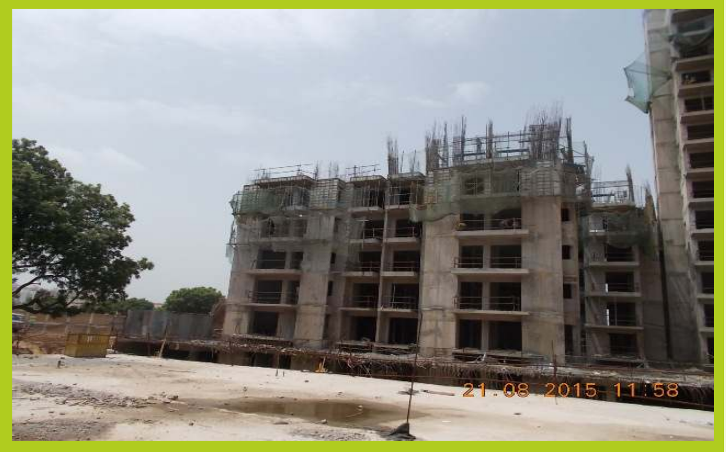
TOWER C August 2015 5th floor slab completed
