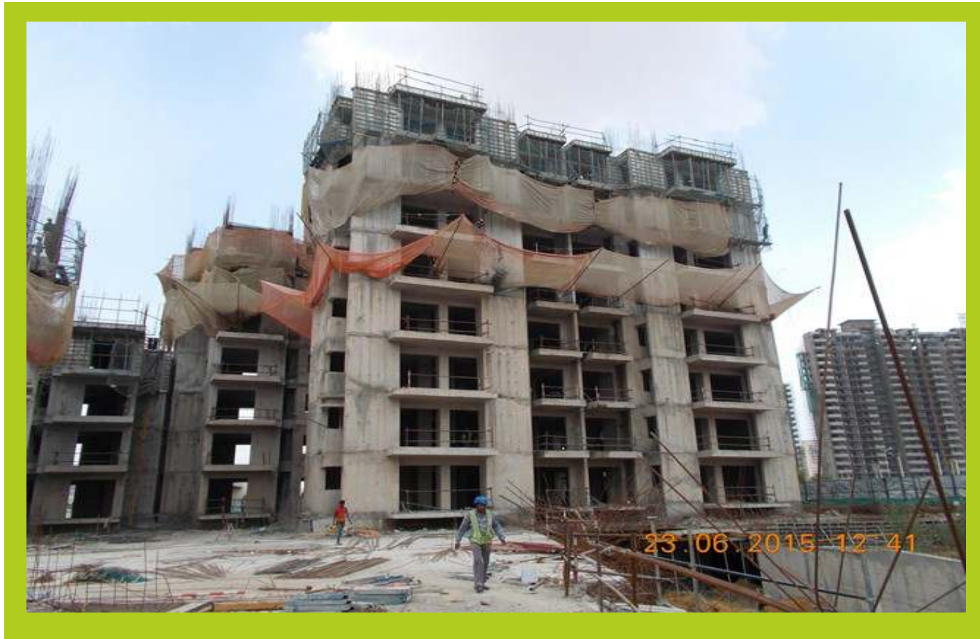
TOWER L June 2015 7th floor slab 67% completed
