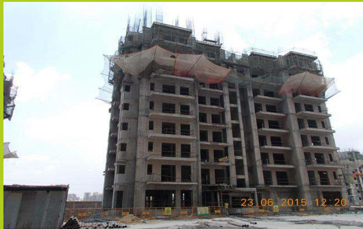
TOWER J June 2015 9th floor slab 50% completed
