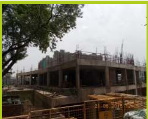
Ground floor slab 80% completed 1st floor slab 40% completed
