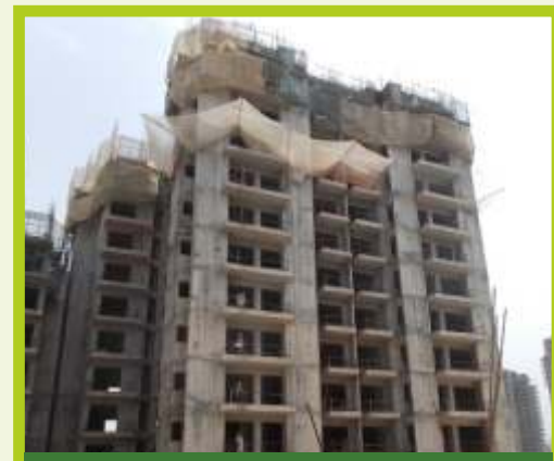
12th floor slab completed
