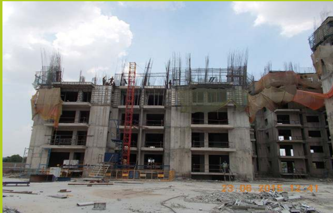
TOWER K June 2015 4th floor slab 67% completed
