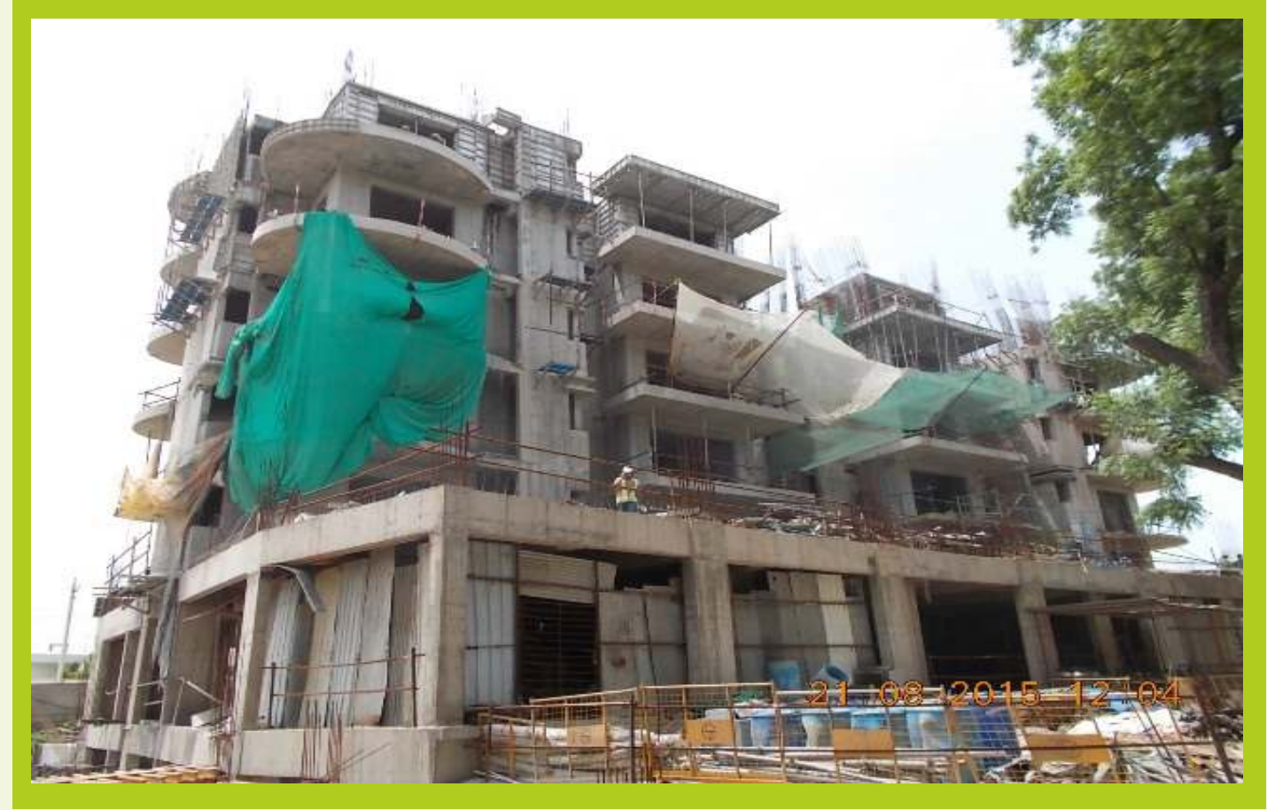
TOWER B August 2015 6th floor slab 50% completed
