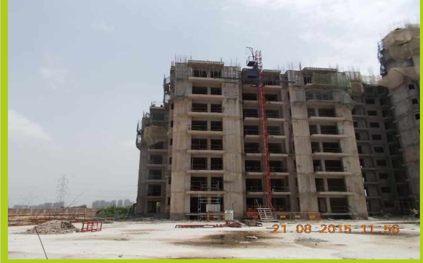
TOWER K August 2015 8th floor slab 55% completed
