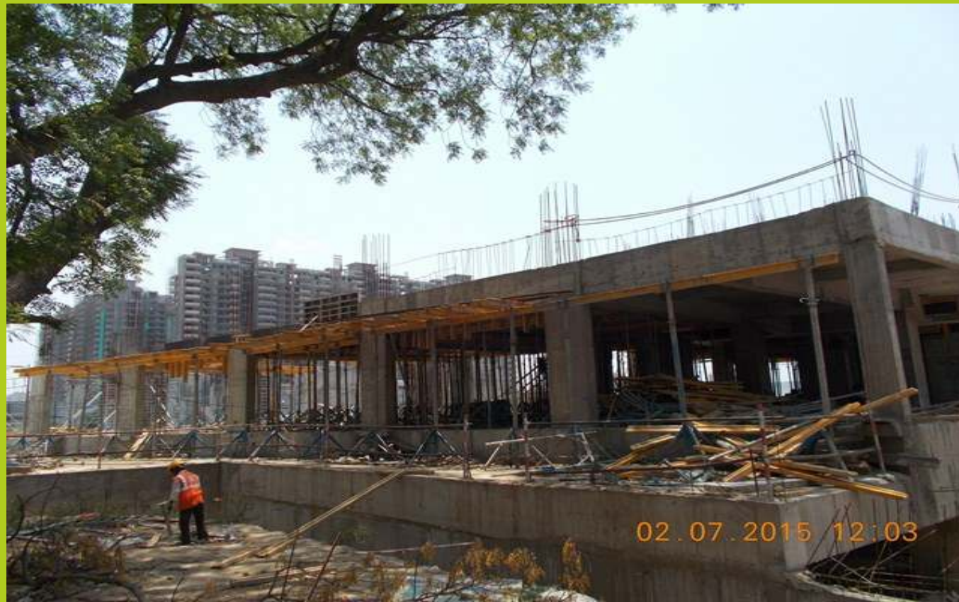
TOWER A June 2015 Ground floor slab 80% completed 1st floor slab 40% completed
