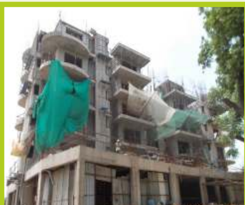
6th floor slab 50% completed
