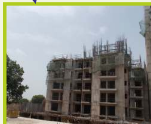
5th floor slab completed
