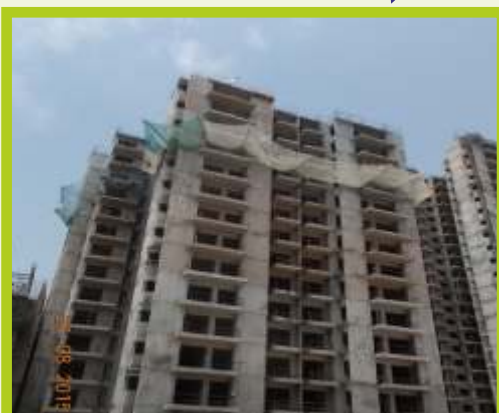
Super structure completed Interior plaster work completed
