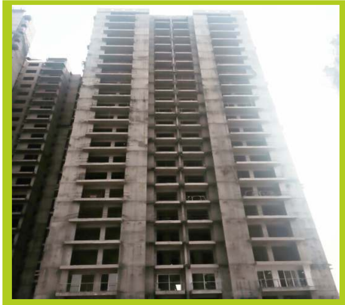
TOWER F June 2015 Super structure completed Interior plaster work under progress
