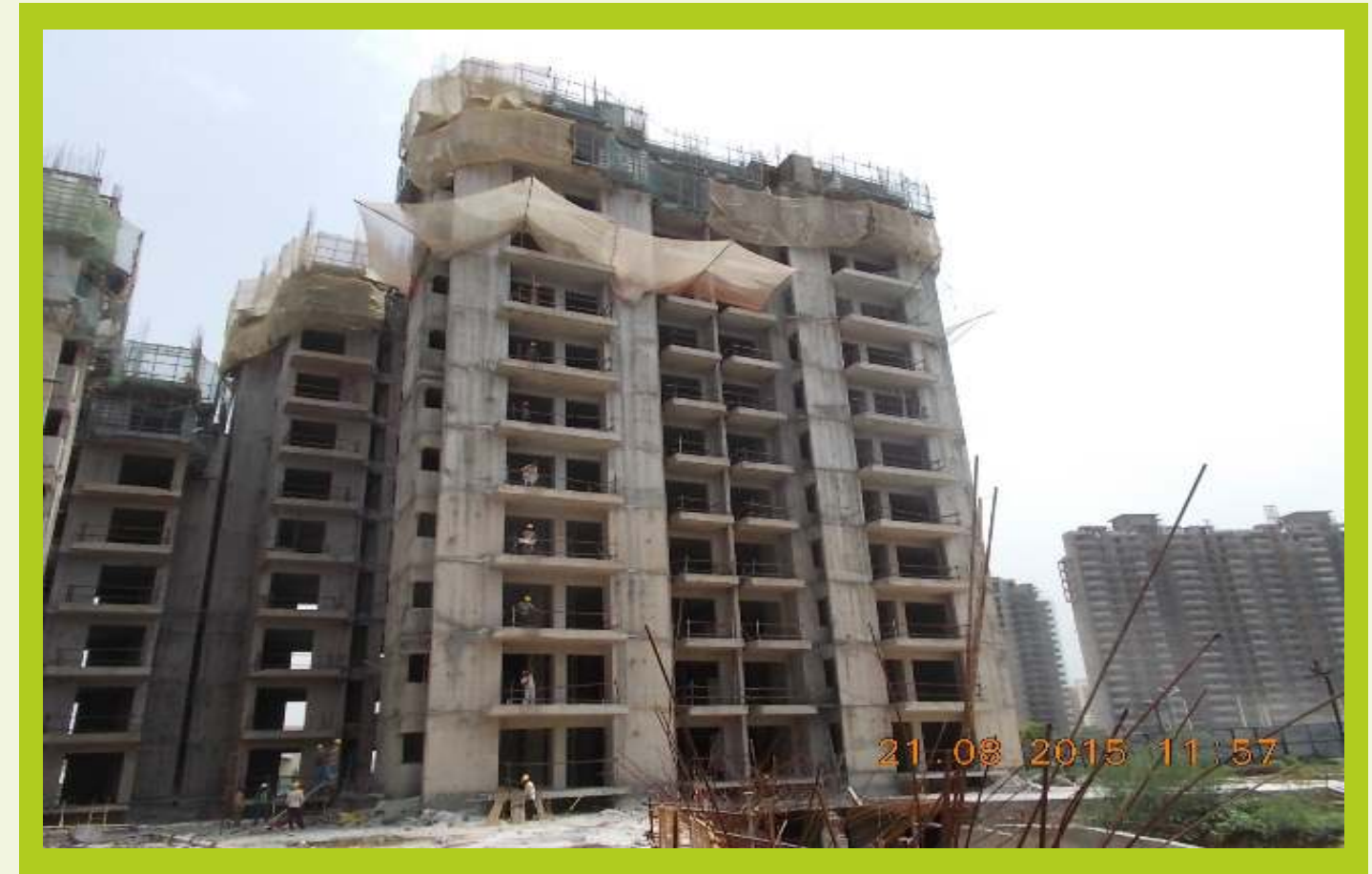
TOWER L August 2015 12th floor slab completed
