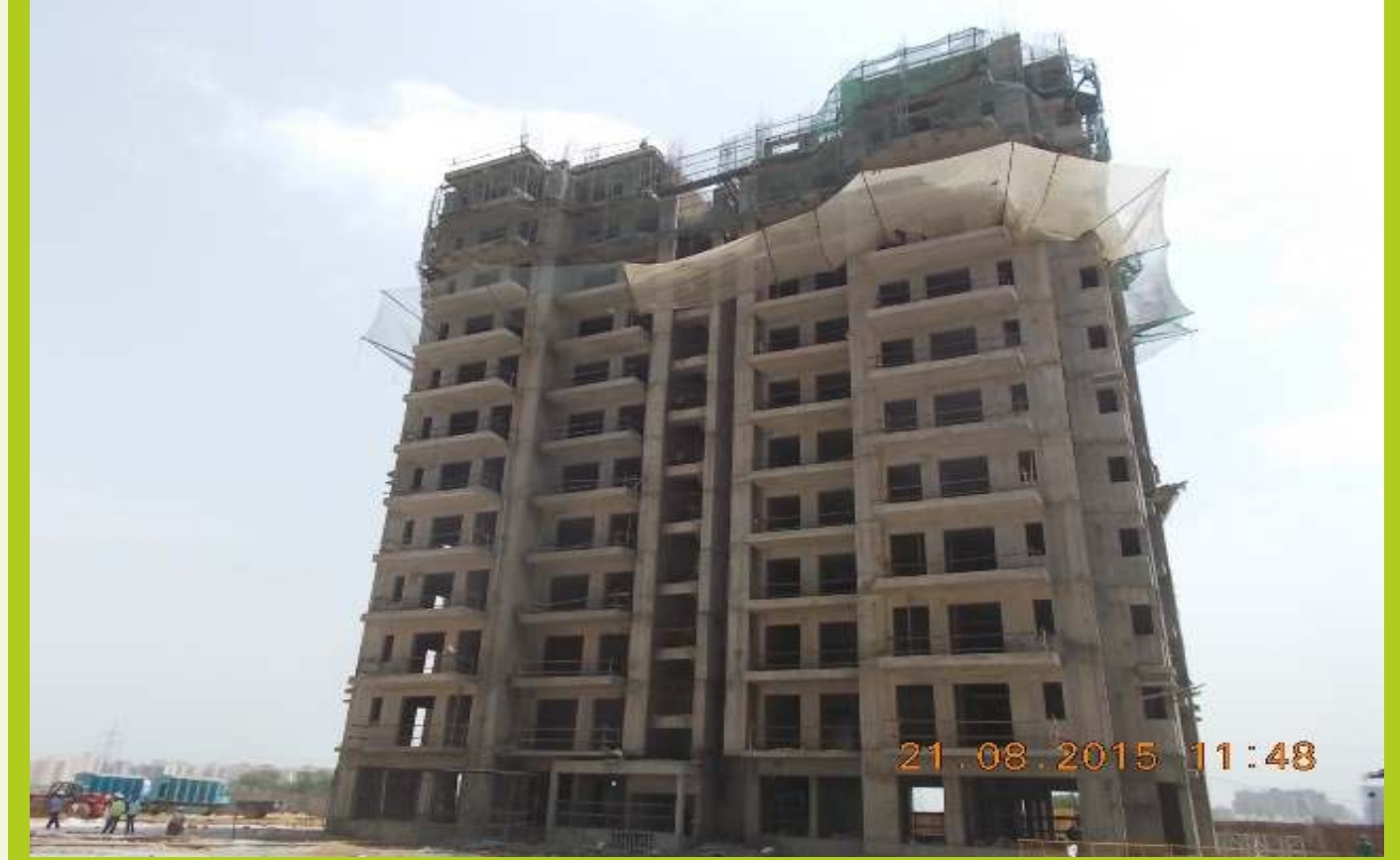
TOWER I August 2015 12th floor slab completed
