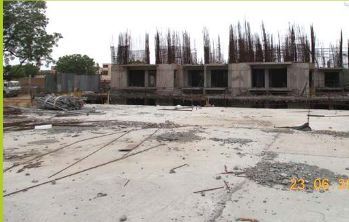
TOWER C June 2015 1st floor slab 67% completed
