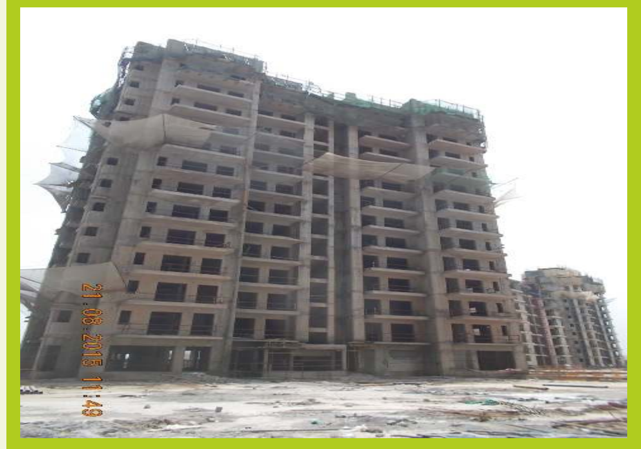
TOWER J August 2015 Super Structure completed
